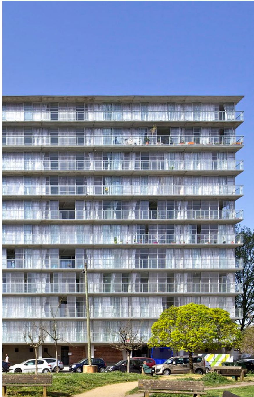
2. Transformation of 530 dwellings— Before and After Lacaton & Vassal, Druot, Hutin
