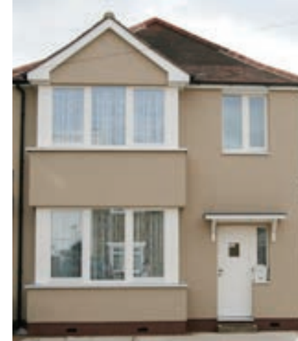
House 109 had external wall insulation and triple glazed windows.
