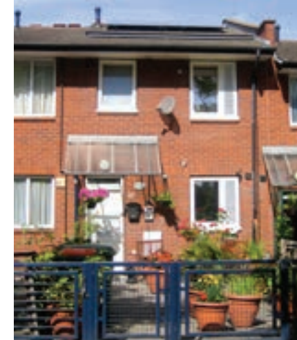
House 8 in London showing the minimal visual impact of the new lightwell in the roof.
